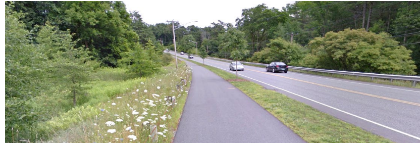
Figure E-1 Multi-use Path along Lyme Road. Source: Google Street View
